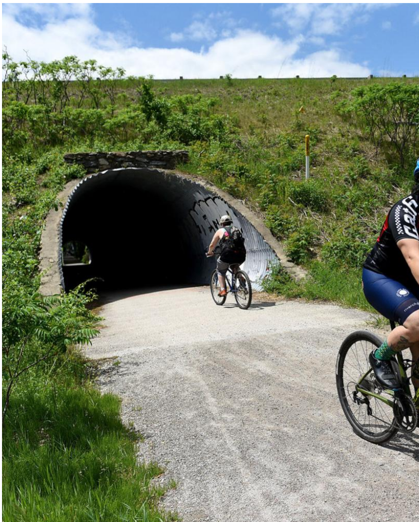
Riders go under the Interstate 93 tunnel on a new section of the Roc DAVID LANE/UNION LEADER
